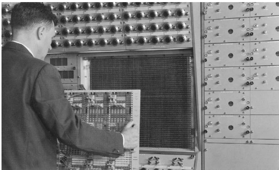
Fig. 3.3. Removing a patch panel from an EAI 231RV analog computer (cf. [EAI PACE 231R, p. 6])
