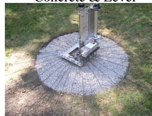
Radial Wires Installed Antenna Installed
