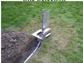
Coax to Base Install Radial Plate Tilt Base & Choke
