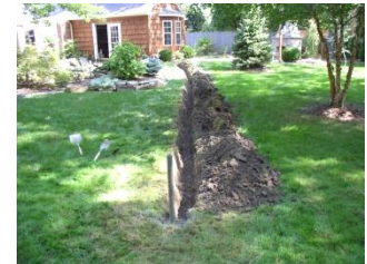
Trench for Coax
