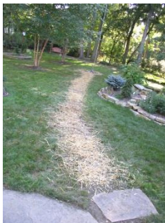
Trench Filled and new grass seeded
